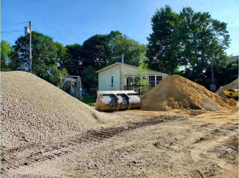
In progress. Image: Community Development Department
