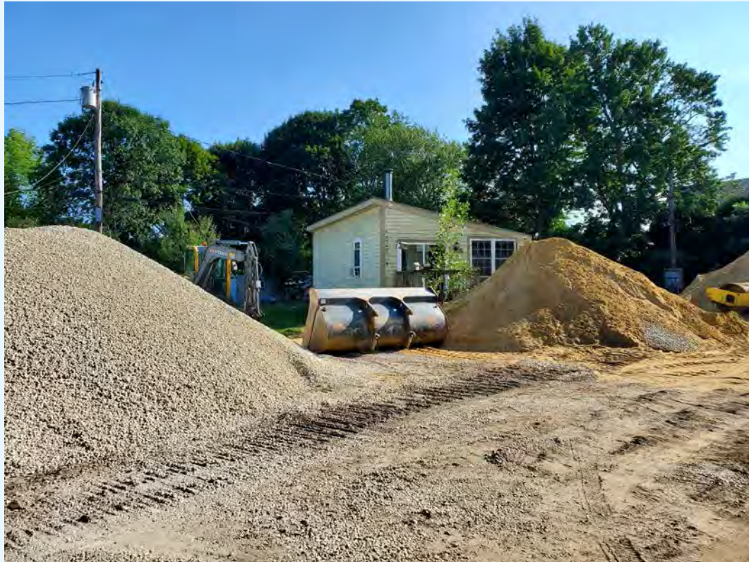
In progress. Image: Community Development Department
